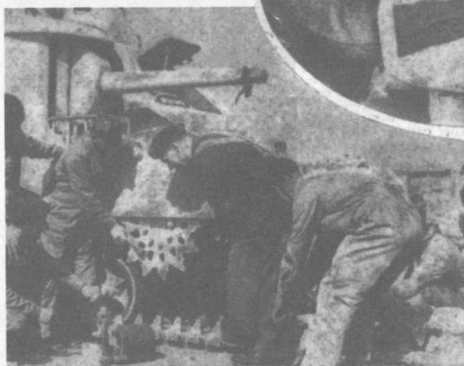
MAINTENANCE MEN of the Royal Tank Regiment removing one of the tracks of a General Grant. Oval , ramming home a shell inside a tank. Right , cleaning the 75-mm. gun. The General Grant weighs about 28 tons and mounts two guns—a 37-mm. and a 75-mm. Though much "boosted" before the battle, after the fall of Tobruk it was stated that the General Grants were already obsolete in America, had vulnerable spots, and were too slow. Certain it was that there were not enough of them.
